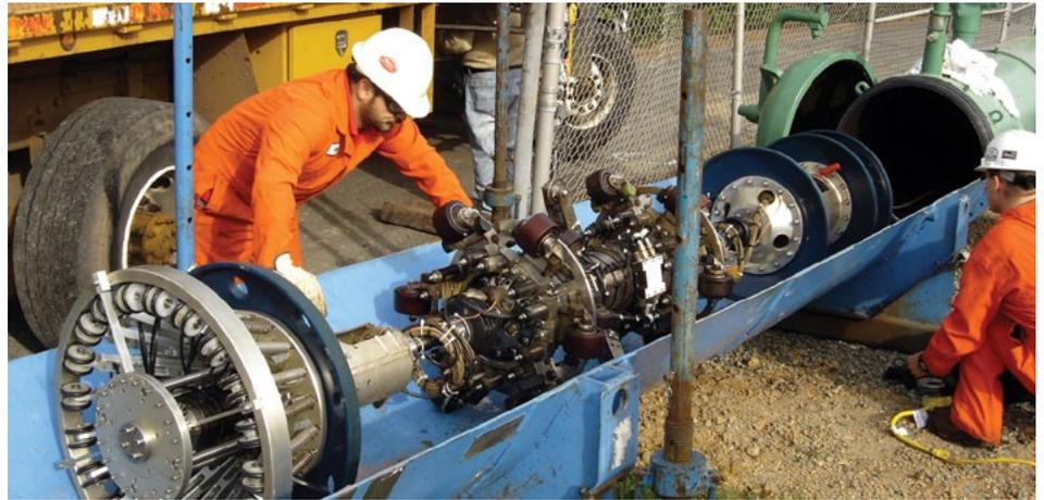
Williams pipeline employees remove an internal inspection device from the pipeline known as a "smart pig."
