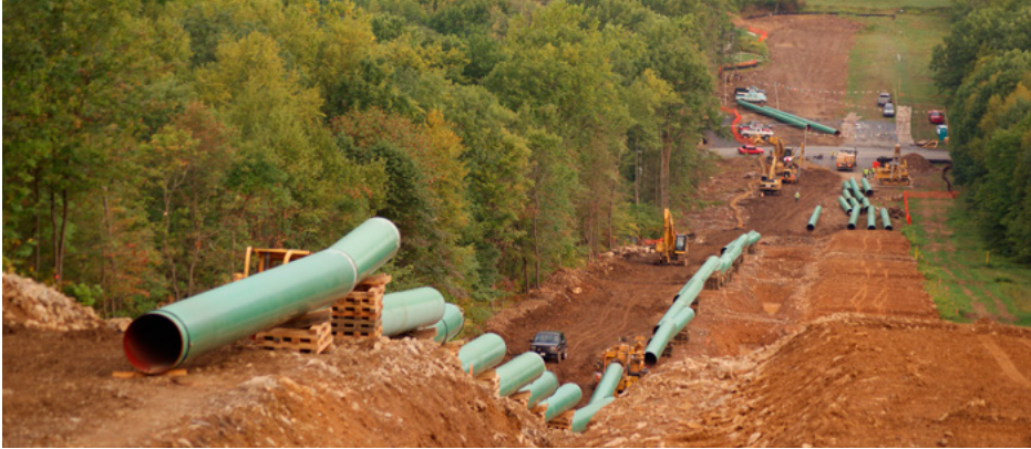
Pipeline construction is anticipated to begin in the spring of 2015.
